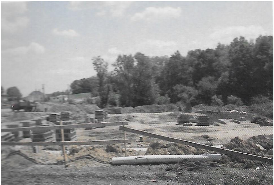
Construction for the 1986 Addition
