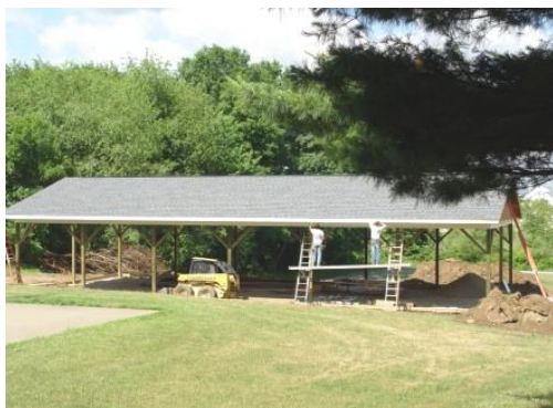
Constructing the New Picnic Pavilion
